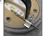
Drill the four mounting screw locations, using the #10 drill bit supplied with screw location fixture.
