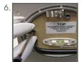
Mount screw location fixture to socket cover using hanger for ring style or latches for ringless style. Rotate fixture to level position. Punch mark the four screw locations.
